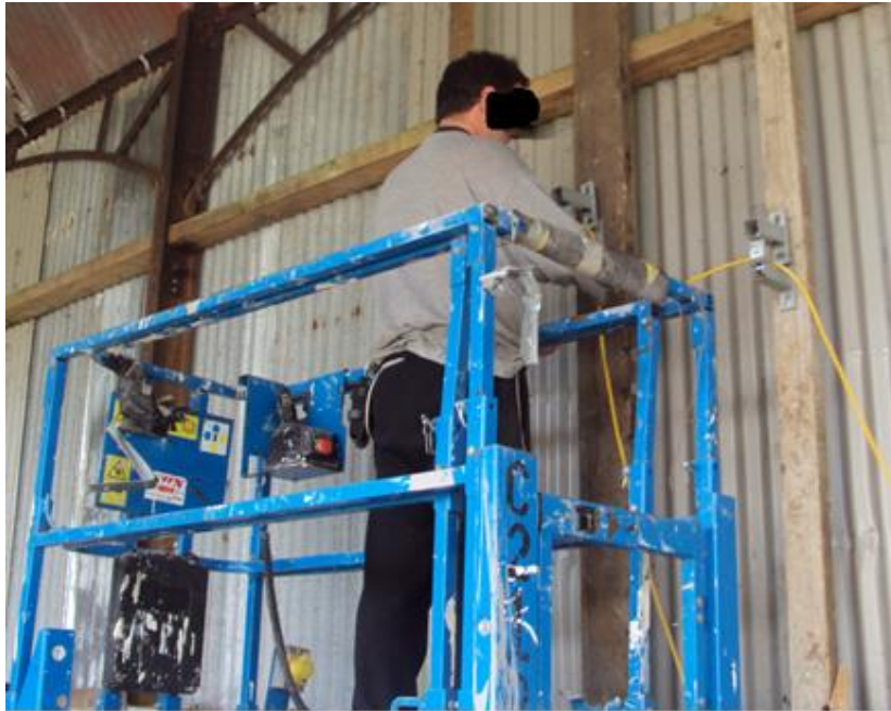
Figure 1 Photo of a participant on the MEWP cabling
